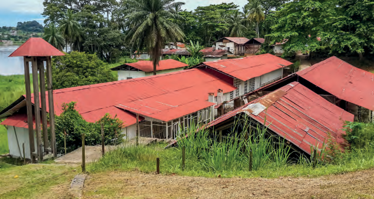
The old Albert Schweitzer Hospital, Lambaréné, Gabon.
